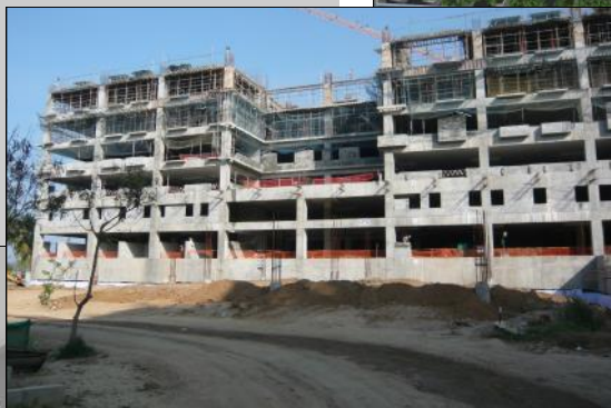
Above: Construction underway
